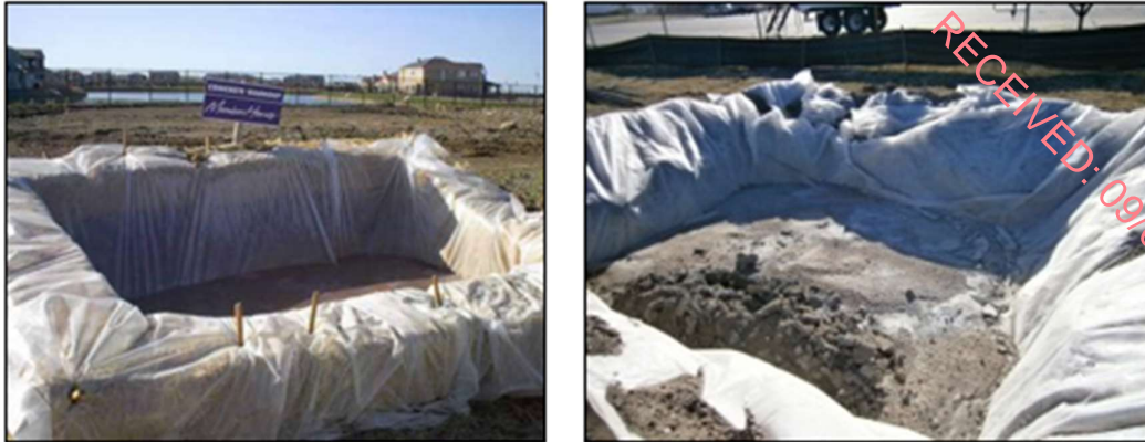
Plate 3-1 Typical concrete wash out areas
