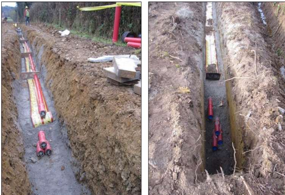
Plate 2-1 Typical Cable Trench View
